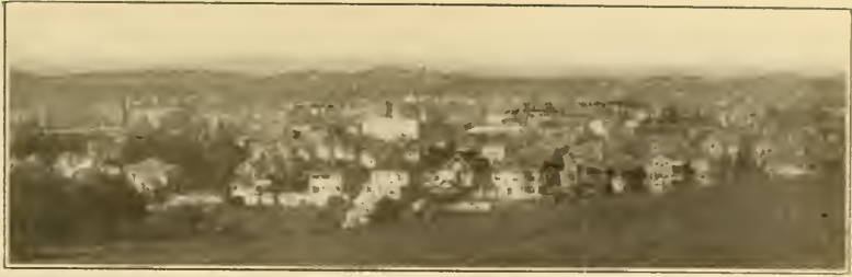
General View of Harrisonburg (Looking North)
