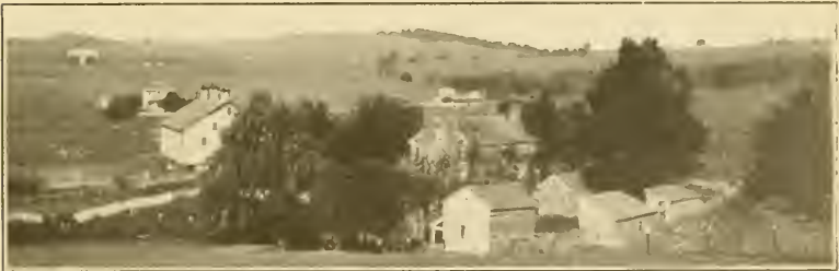
Log House in Center, First Postoffice in Rockingham (Page 212)
