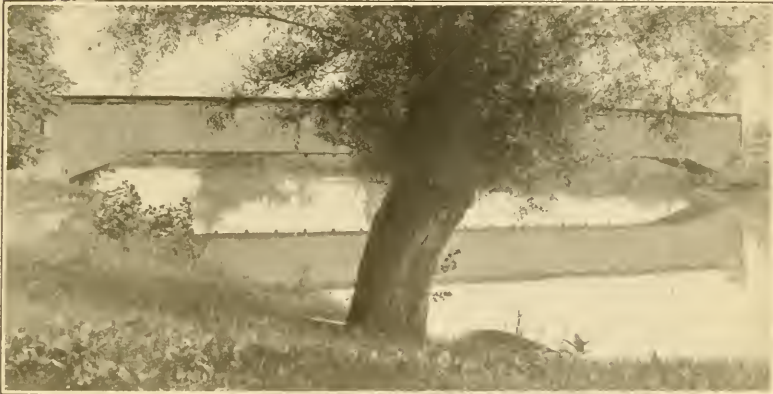
The Bridge at Bridgewater
