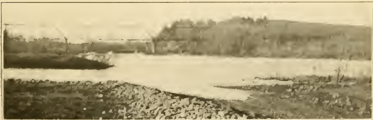
Port Republic: Confluence of the Rivers, the Bridge, and the Heights toward Cross Keys
